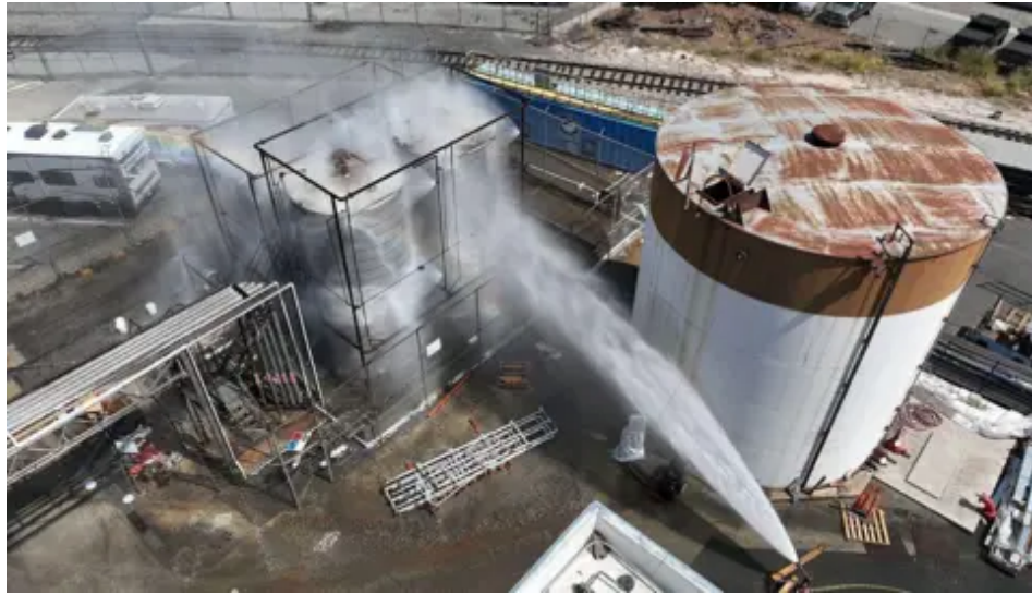
3 4 5 6 7 8 9 10 11 12 Figure 1: Firefighters Cooling Tank
